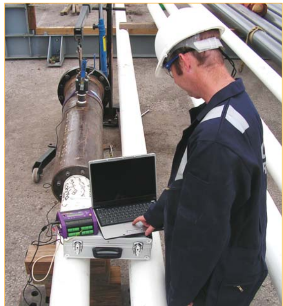
Pressure data is logged during the PIGGING process
