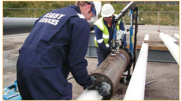
The PIG receiver being bolted into place
