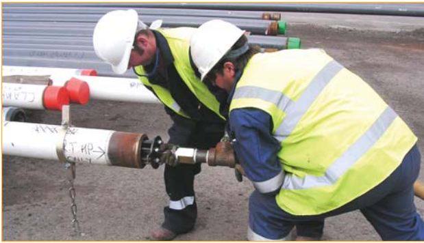
The launcher being connected to a 750cfm compressor
