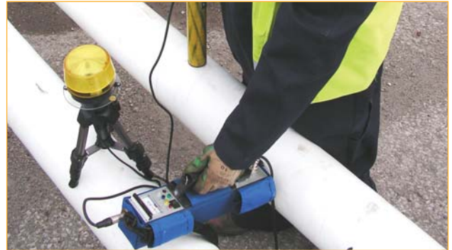
PIG tracking being carried out on an above ground pipeline
