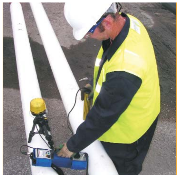
PIG tracking being carried out on an above ground pipeline
